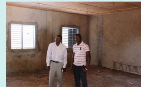
End of August - Roof is on, doors and windows in. Waiting to be decorated and filled with desks!
