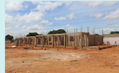
June - The walls start going up.
